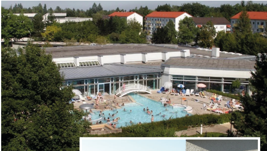
Pullach swimming pool heated by deep geothermal
